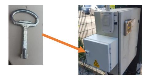
The switch turns off all power to the gates and will disengage the magnetic locks
